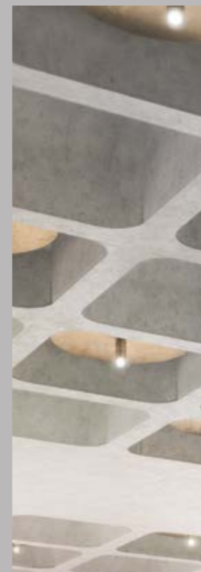
RESTORED ORIGINAL SOFFIT
