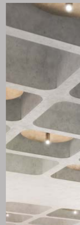
RESTORED ORIGINAL SOFFIT
